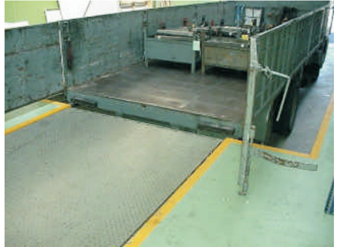
Leveller fully lowered
