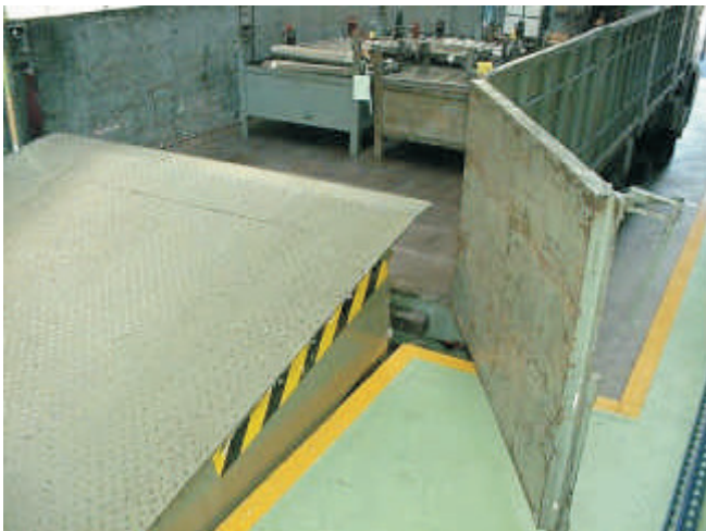
Leveller lowering with lip extended
