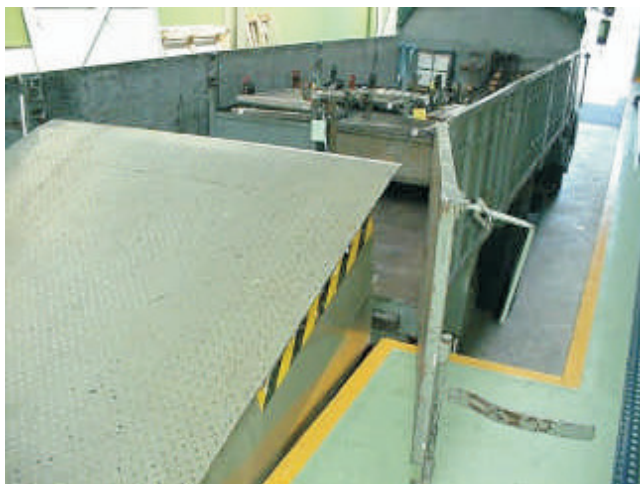
Leveller in rest position - doors open
